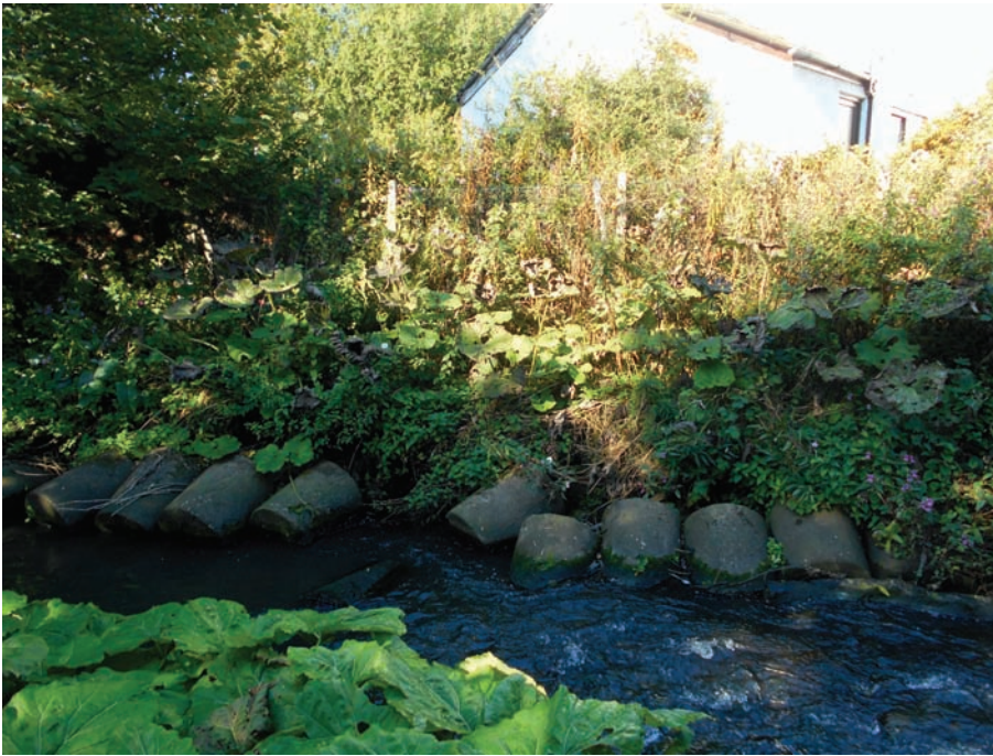
Figure 4: The Irk at Chadderton in 2015 showing concrete blocks reducing erosion on the north bank upstream of Street Bridge.
