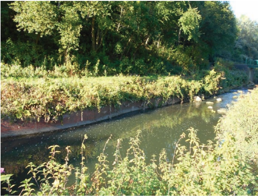
Figure 6: Brickwork installed to stabilize the channel of the Medlock at Clayton Vale.
