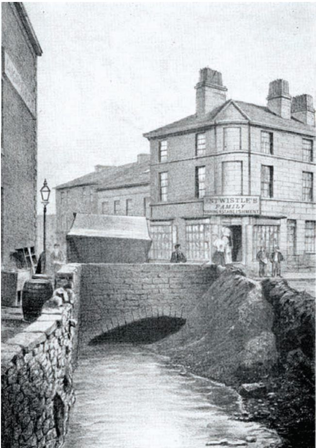
Figure 14: The 19 th century River Irwell at Bury where debris thrown into the river has left little room for high flows to pass under the bridge.
