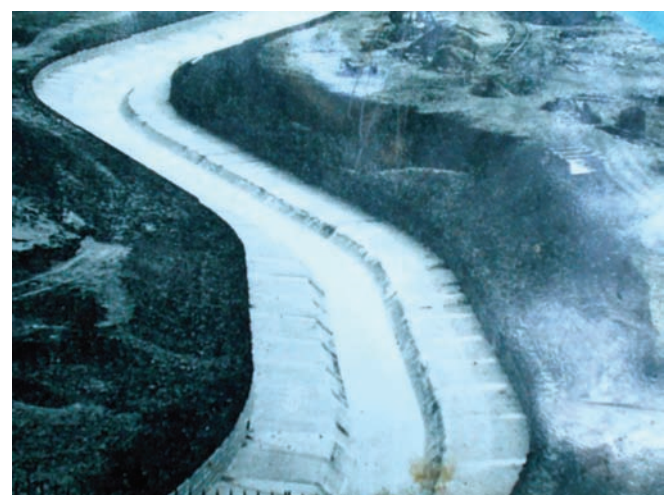
Figure 7: Photo of a picture of the double trapezoidal channel created in 1909 for the River Medlock round Philips Park and the Cemetery (from an information panel at Clayton Vale).
