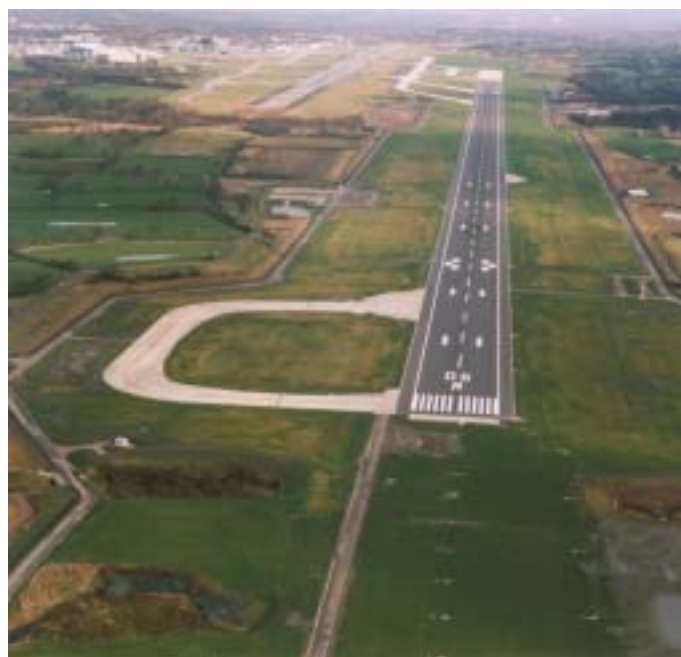
Figure 1: An aerial view of Runway 2 looking north east.
