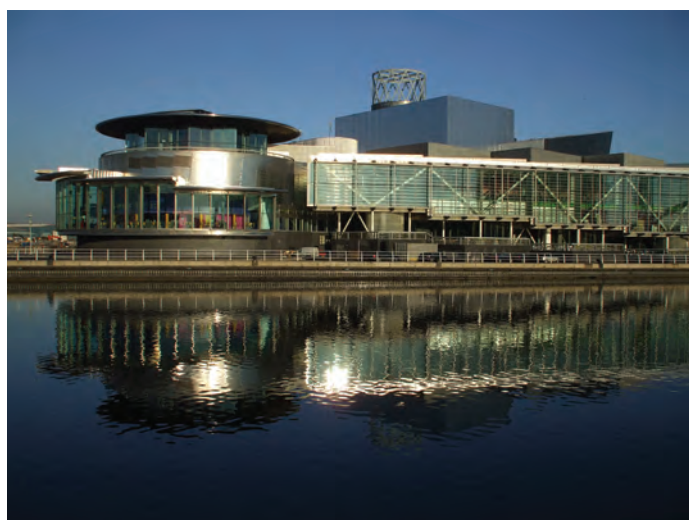
The Lowry: site 7.
