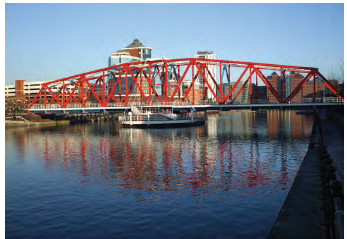
Detroit Bridge, site 6.
